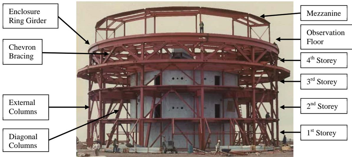
Figure 5: CFHT enclosure pier steel frame during construction
