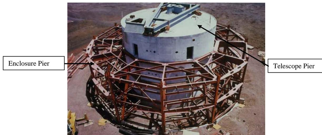
Figure 3: Telescope pier building and enclosure during construction
